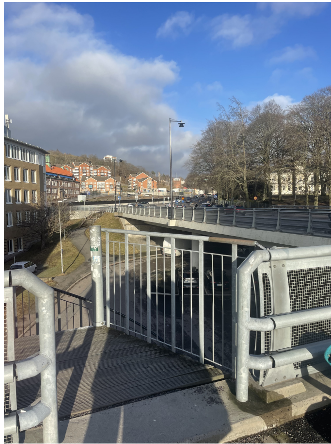
Figure 4.13: The spiral staircase at Mölndals bro, which respondents point out as a hindrance.
