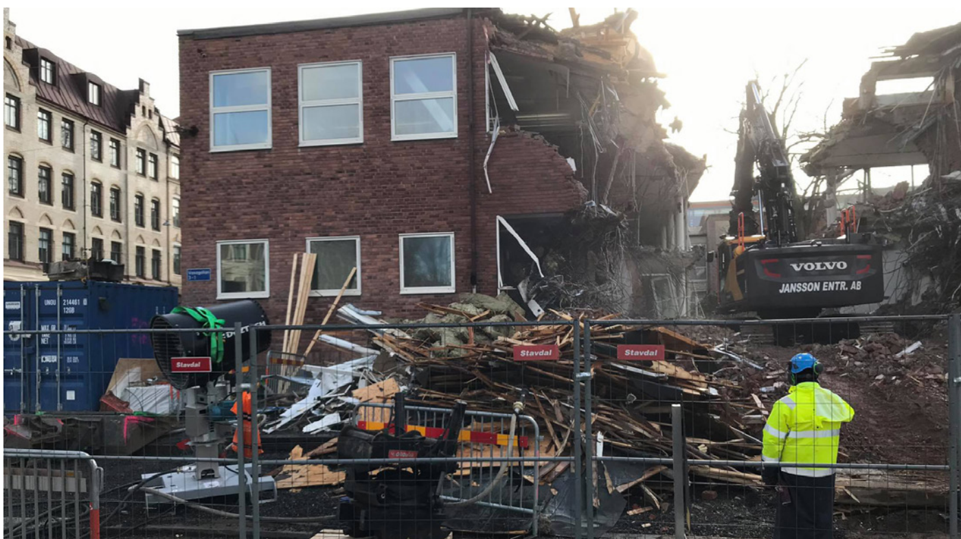
Picture 1 and 2. Demolition site, Handelshögskolan in central Gothenburg, source: authors
