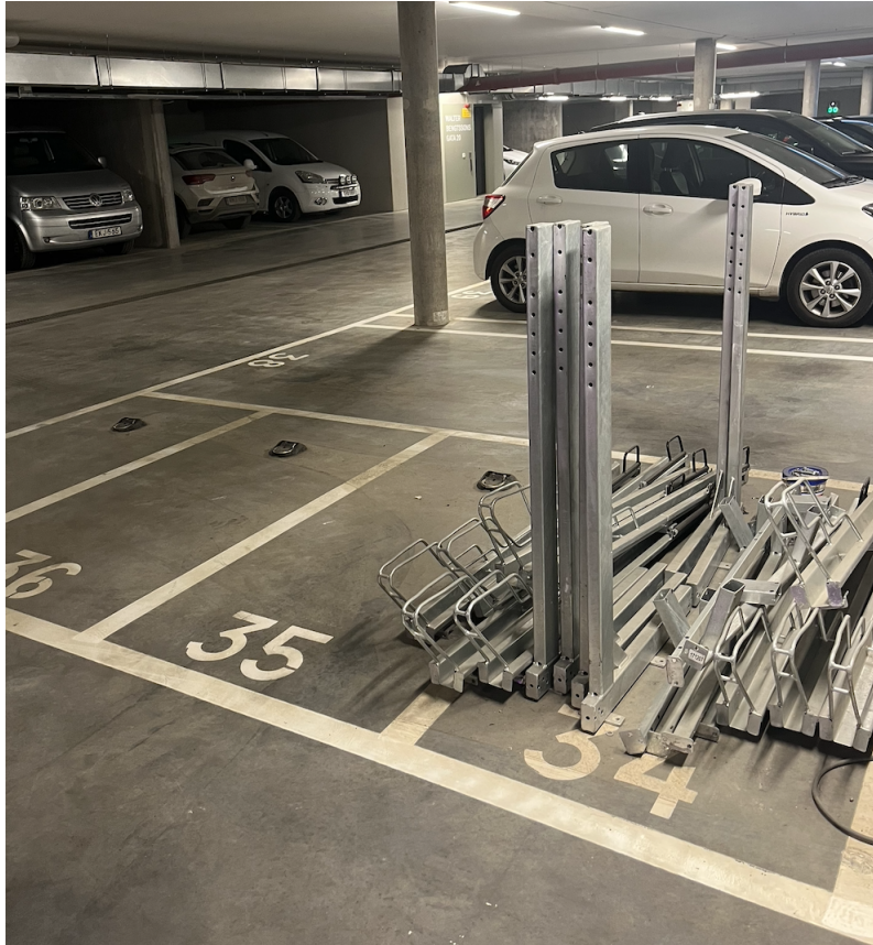
Figure 7.7: An uninstalled two- tier bicycle rack in one of Fixfabriken garages.
