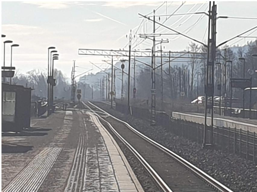
**Figure 4.10:** Photo of the railway track at Lindome station. It is possible to see how the railway tracks and platform form a slope after the tunnel.
