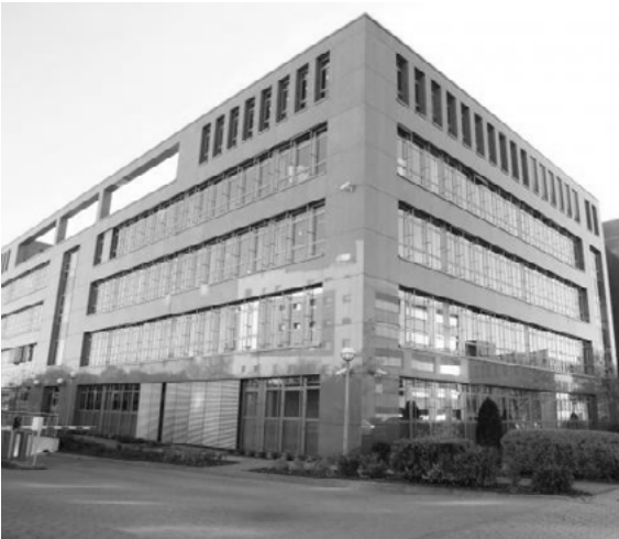
Figure 15: Existing façade of Da Vinci Source: Author
