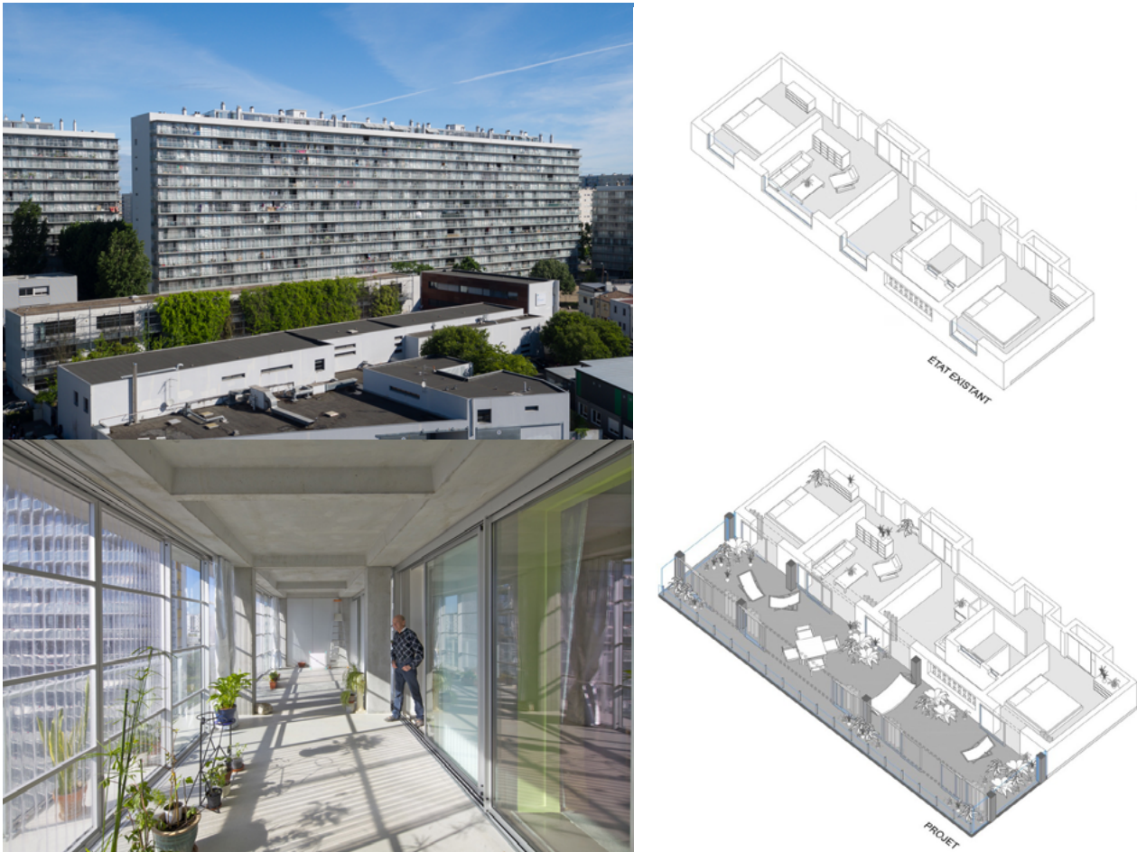
Figure 45: Grand Parc Bordeaux Source: Lacaton & Vassal, 2017
