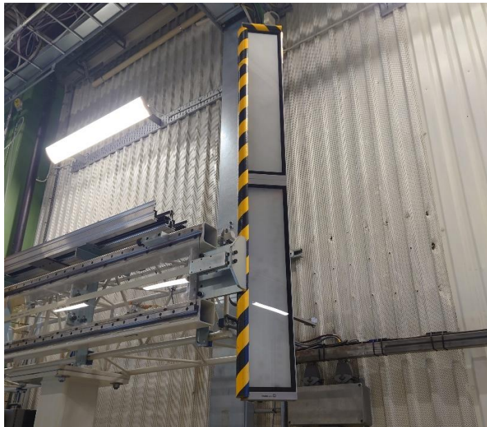
Figure 20 – Lights used for creating good lighting conditions
