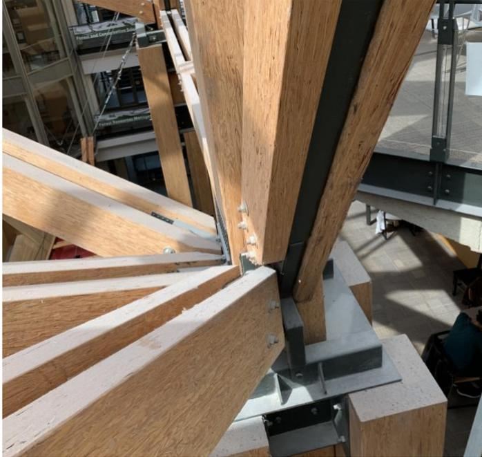
*Figure 2.4 Complex steel connection between timber elements.*
