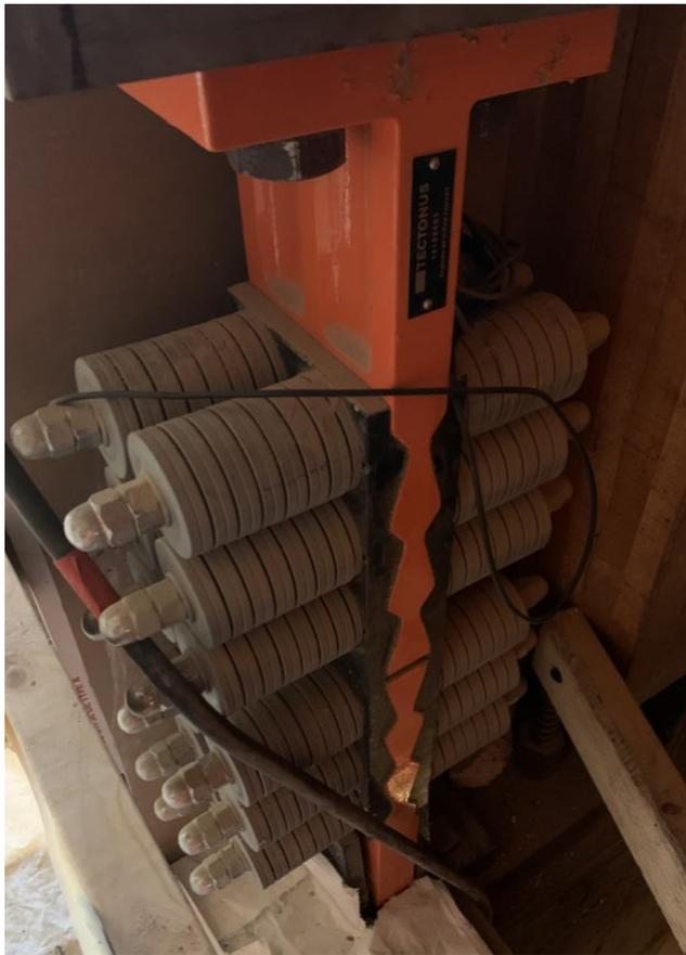
*Figure 5.7 Example of an energy dissipation device.*
