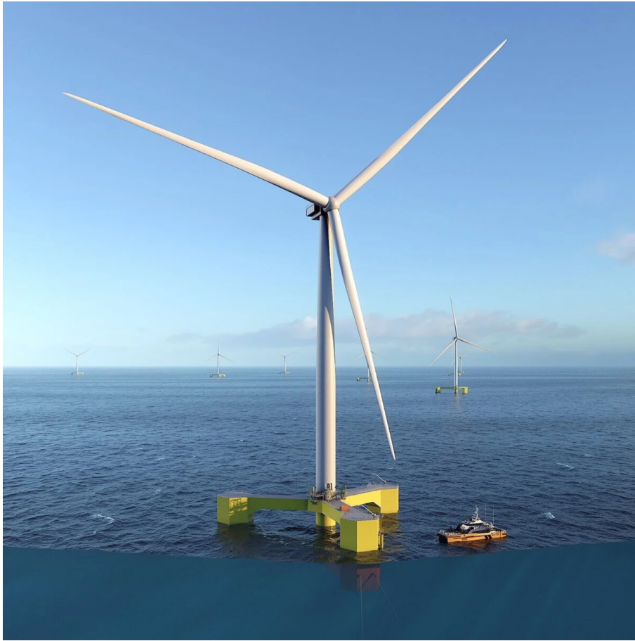
Figure 1.2: The Semi-submersible FOWT YFloat TM [19].
