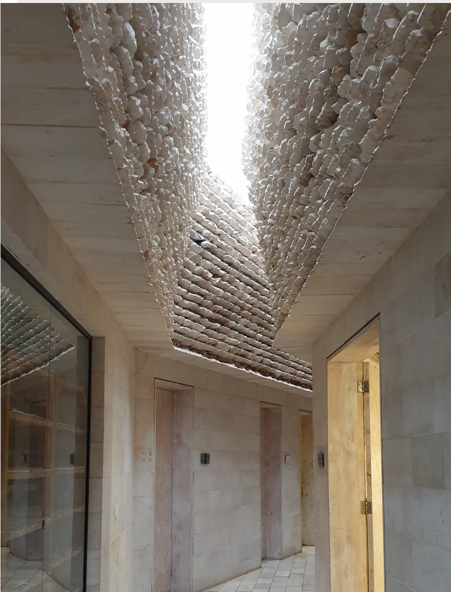
Ajloun Royal Academy for Nature Conservation , located on the borders of Ajloun natural reservation, built by RSCN and Designed Architect Ammar Khammash
