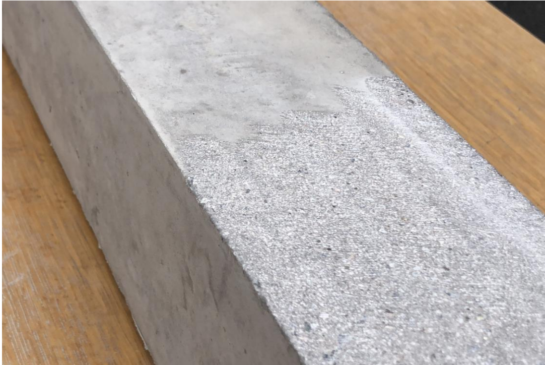
Figure 8.6 Example of grinded surface compared to ungrinded surface.
