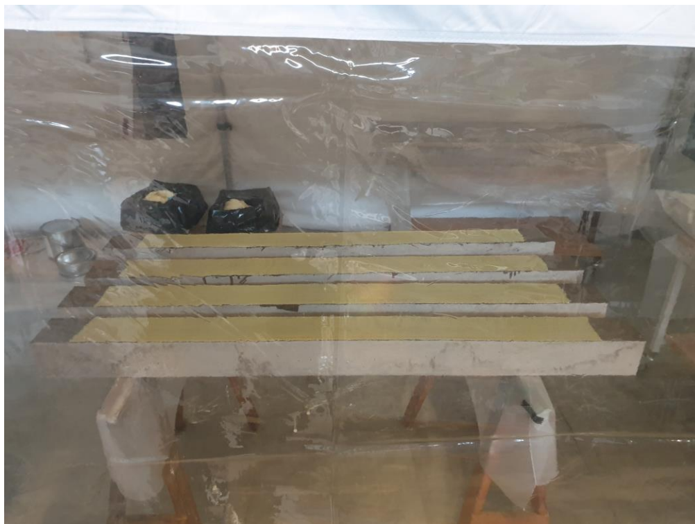
Figure 8.11 FRP attached to the concrete surface.
