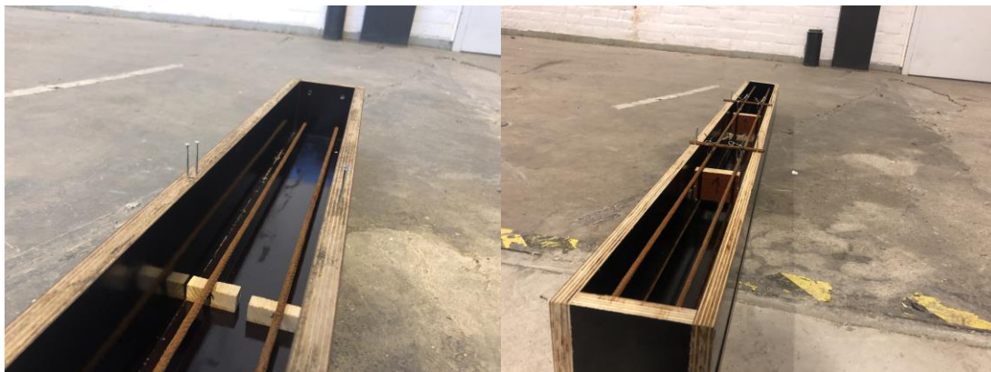
Figure 8.2 Placement of reinforcement.
