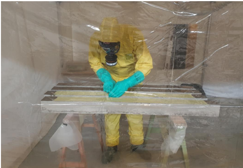
Figure 8.9 Application of adhesive and FRP to the bottom surface.
