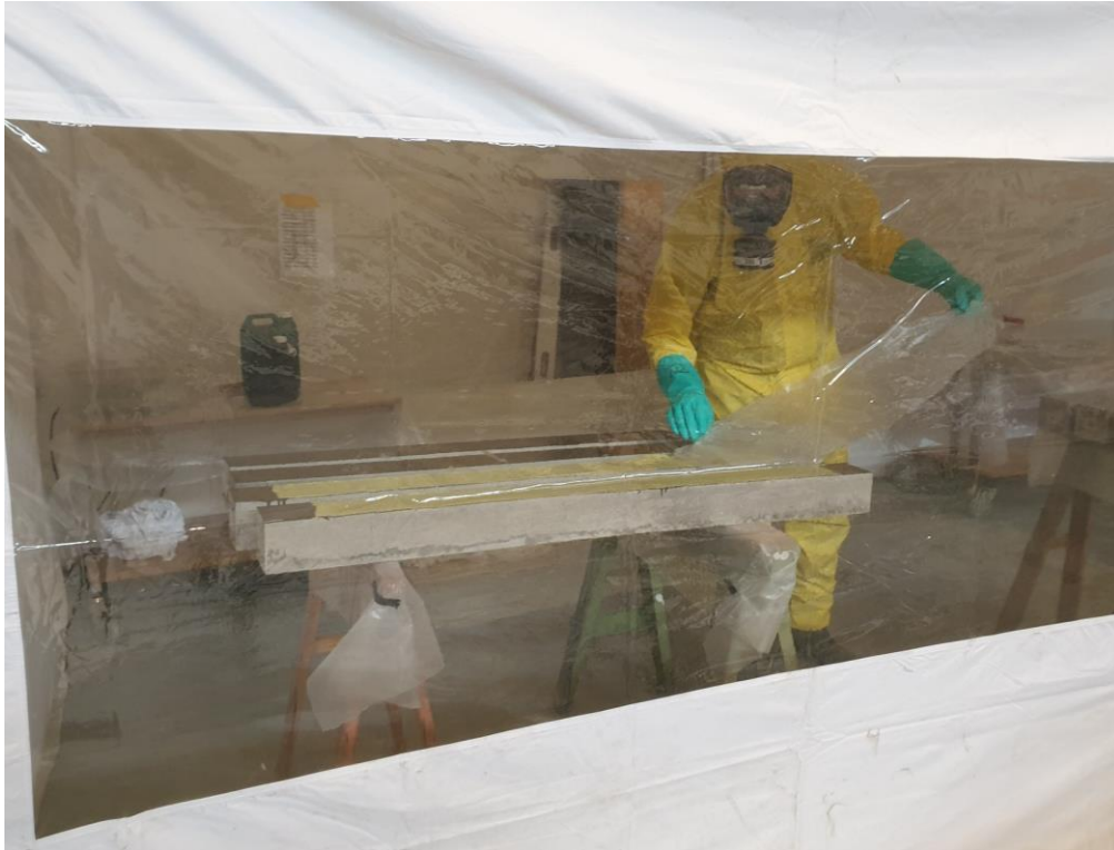
Figure 8.10 Application of adhesive and FRP to the bottom surface.
