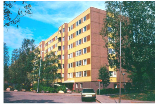
Figure 32: The original facade
