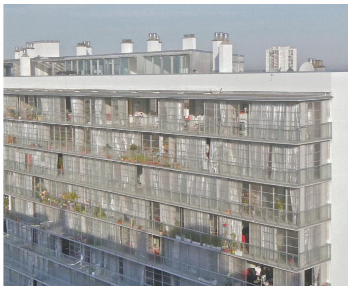
Figure 21: The new facade
