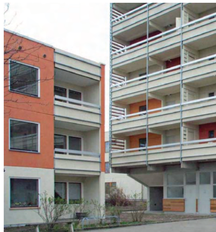
Figure 15 & 16: The building facades before and after the renovation
