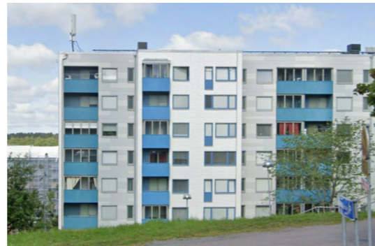
The facade after the renovation
