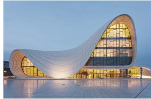
Structure is totally hidden under the curved plate when the building is completed.
