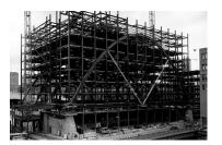
3.3 Horizontal thrust balance the bending forces and compression in semi-circle arch
