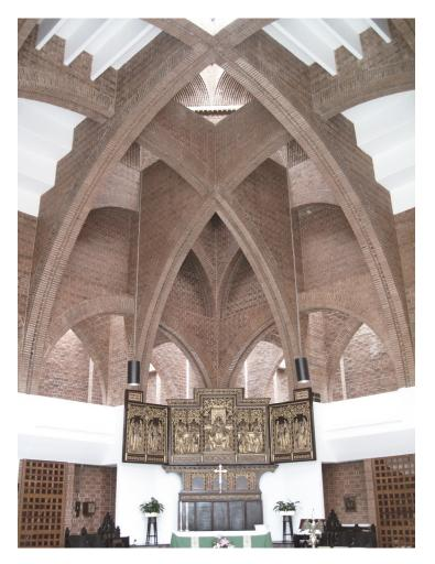
Interior scene of christ church shows that it is a structure dominate space. The double arches cross with each other and sketch the outline of interior space. Half arches hold the main structure and diffuse the daylight.
