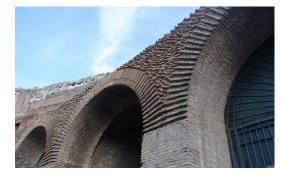
The reinforcement masonry and the semi-circle arches in Colosseo, Roma, Italy
