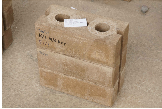
Figure 7.13: Series C7 - dry stacked triplet without keys showing no damage after testing.
