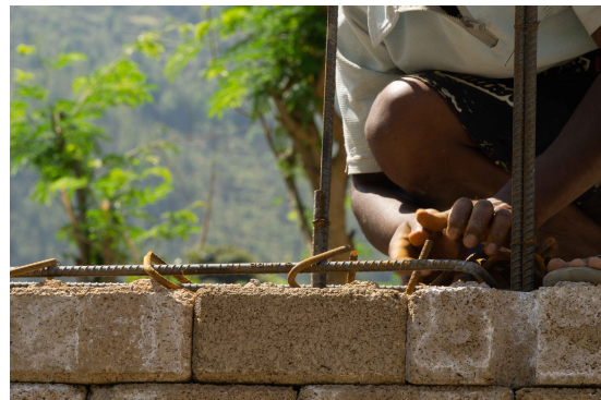
(b) Rebar preparation for lintel band.
