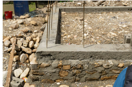
(b) Foundation and plinth band cast with vertical rebar sticking up.
