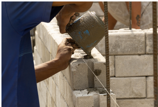
(a) Grout pouring in CSEB voids.
