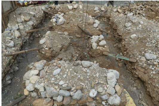
(a) Foundation dug out of house. Vertical rebar prepared for anchoring.
