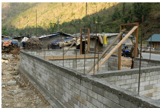
(c) Casting of sill band.
