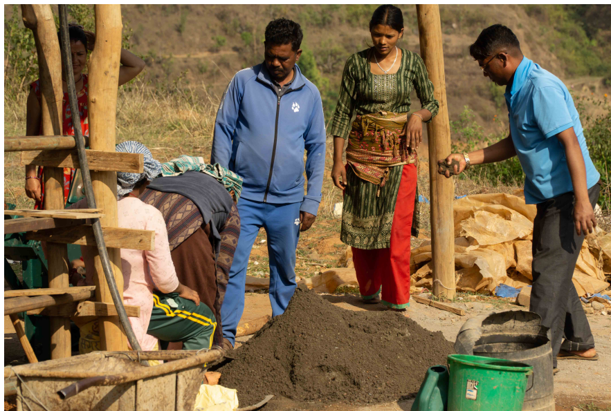
(c) Soil, sand, cement and water mixing.
