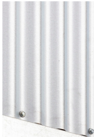
Sinus corrugated galvanized steel façade and roof
