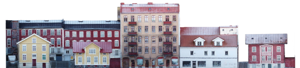
Elevation by drone photogrammetry April 2022
