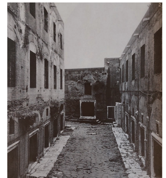
above. image 4 Höjdgatan Landala around 1967 before demolitions below. image 5 Trajan's stables Via Baberatica 110 ad.
