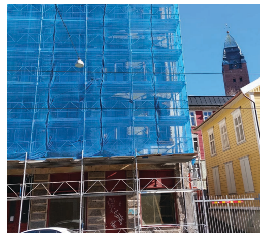
Renovation on Bangatan 10, March 2022
