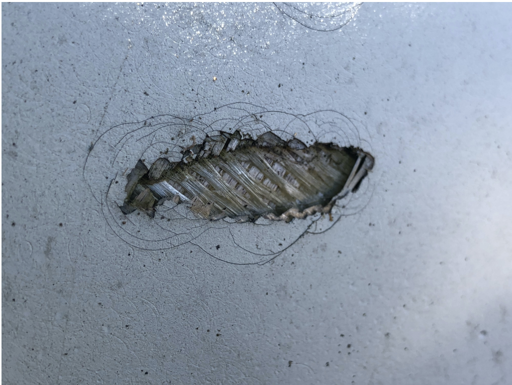
Figure L.5 Damage of leading edge with visible glass fibre weave (own photo).
