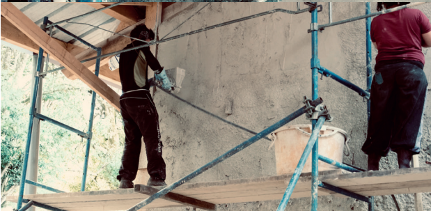
Rush shots: Construction of the barn
