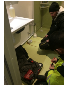
Remove WC and Plugging the sewage
