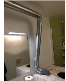
Plugging in on existing ventilation
