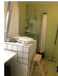
Finished recycling toilet
