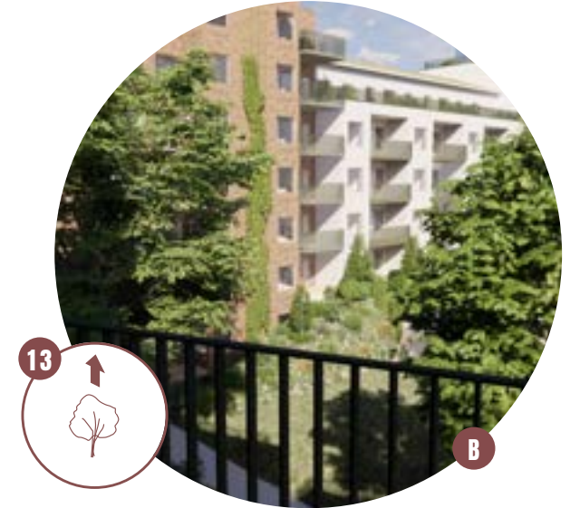
Fig 78. Vegetation on walls and big trees makes nature present on all floors in the buildings.
