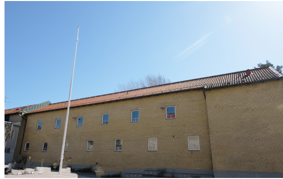
Figure 28: West facade of school 2
