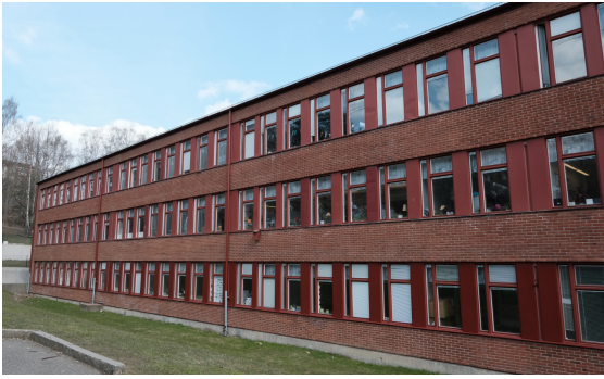
Figure 27: West facade of school 1
