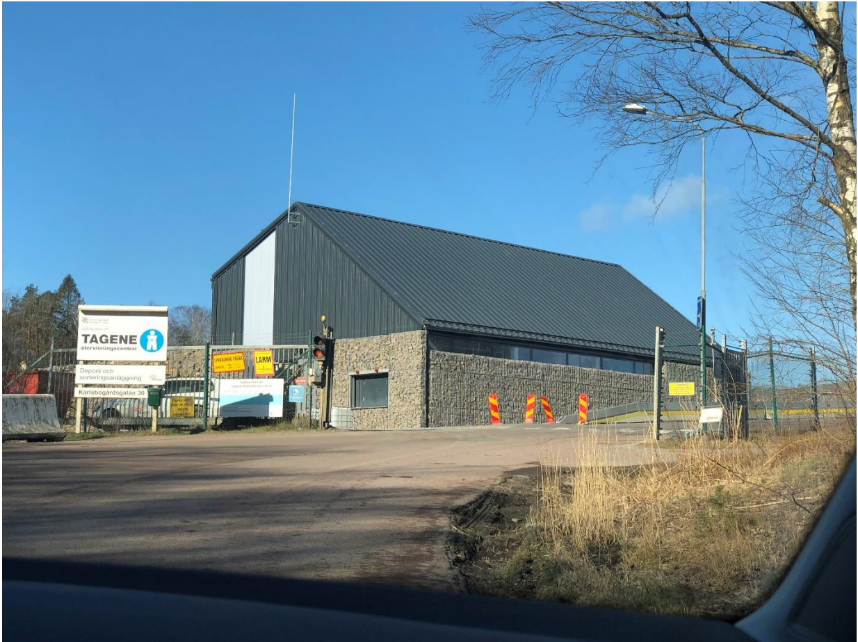
Figure 17: A new building that is found at Tagene, with a roof orientation towards north east.
