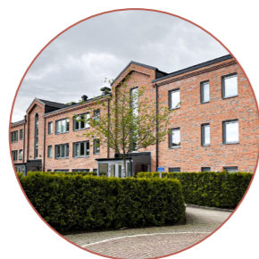
RESIDENTIAL BUILDING ON KORTEDALA TORG BUILT 2015
