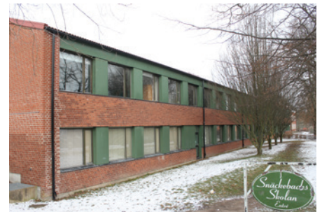
c. Rhythm and repetition, horizontality, bricks and greenish metal cladding.
