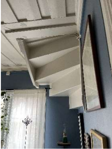
Figure 10 The stairs leading to the attic are visible in the living room.
