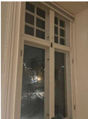
Figure 17 The large windows that provide plenty of light.
