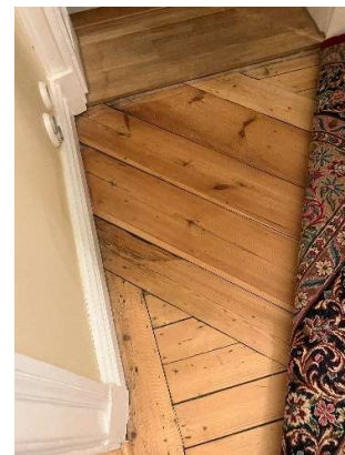
Figure 24 You can see where the fireplace in the bedroom has been.
