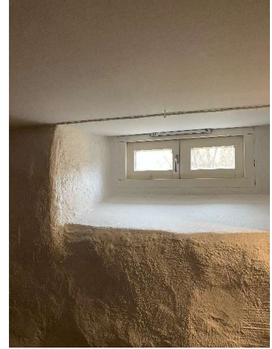
Figure 12 The basement has thick walls and small windows that still let in a lot of light.
