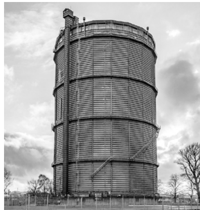
Gasklockan at the Gullbergsvass gasworks, Gothenburg.
