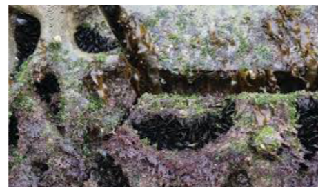
Figure 7.6. Living seawall from Sydney Harbour
