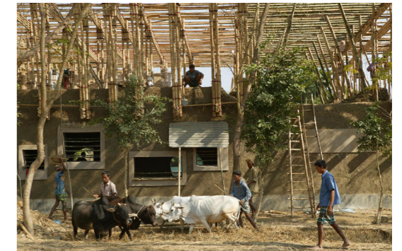
Figure 7.10. Building process of the METI school
