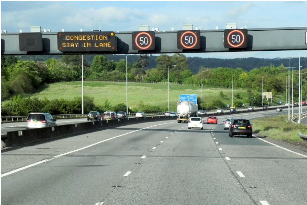
Figure 3.1: Overhead gantry sign combining VMS and VSL (David Dixon, 2013)
