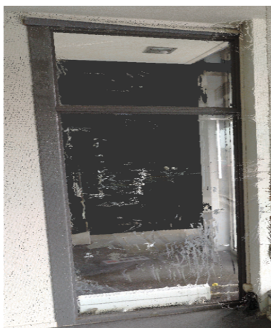
Figure 7: Entrance window (3D-scanner)
