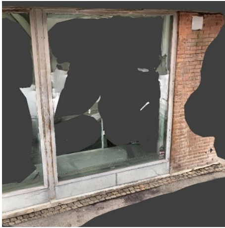
Figure 19: Facade Window (Scaniverse)
