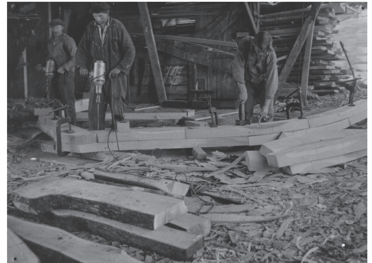
Fig. 33. Assembly of frames for a new boat at J.W. Bergs yard
