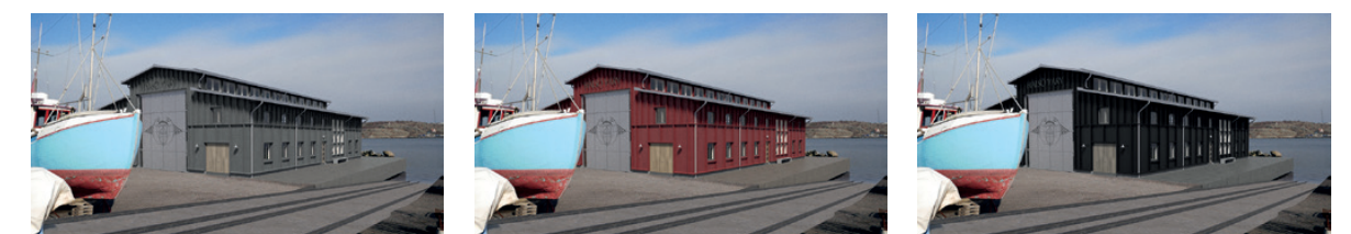
Fig. 65. Testing different facade treatments. Gray tar vitriol, Falu red paint and Falu black paint
