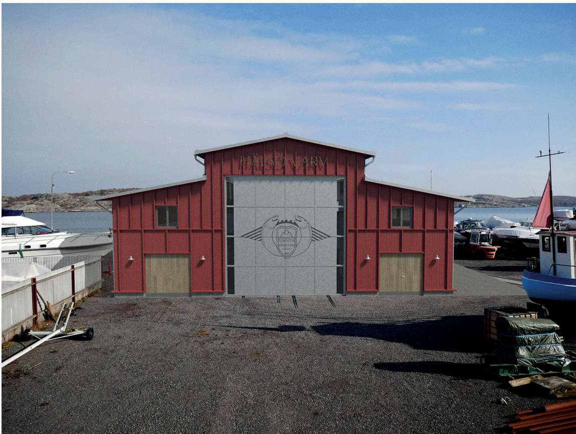
Fig. 89. View from west
