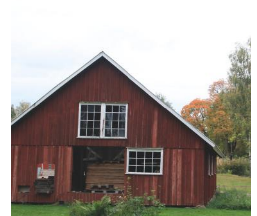
Fig. 34. Former sawmill, Strömsfors, 2022
