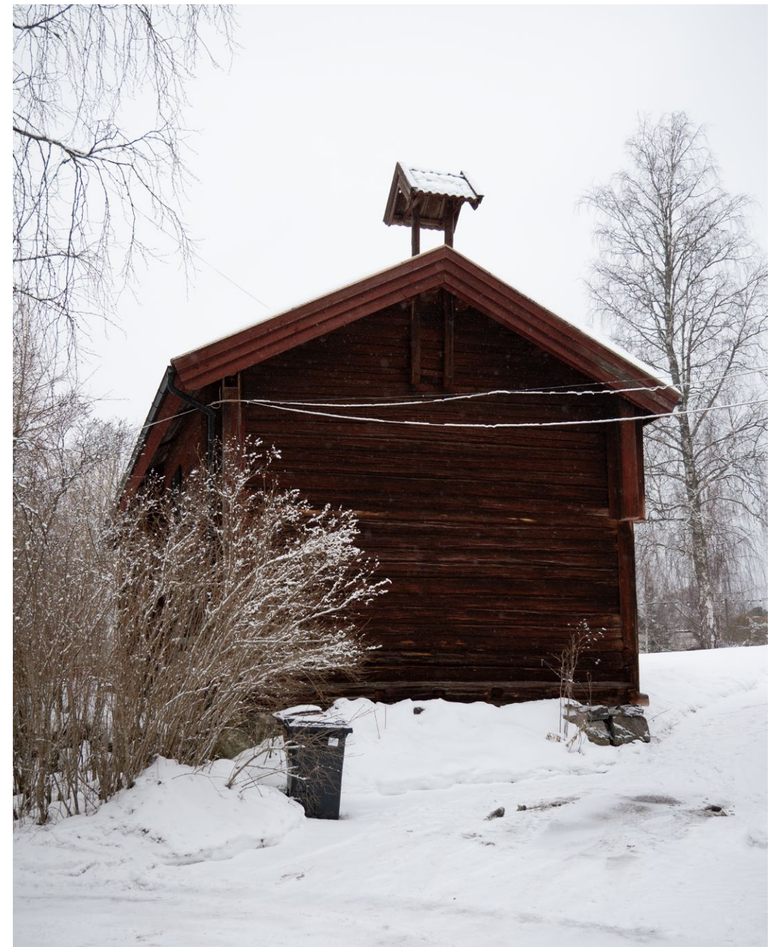
Fig 20. Storage building in Stora Hyttnäs.
