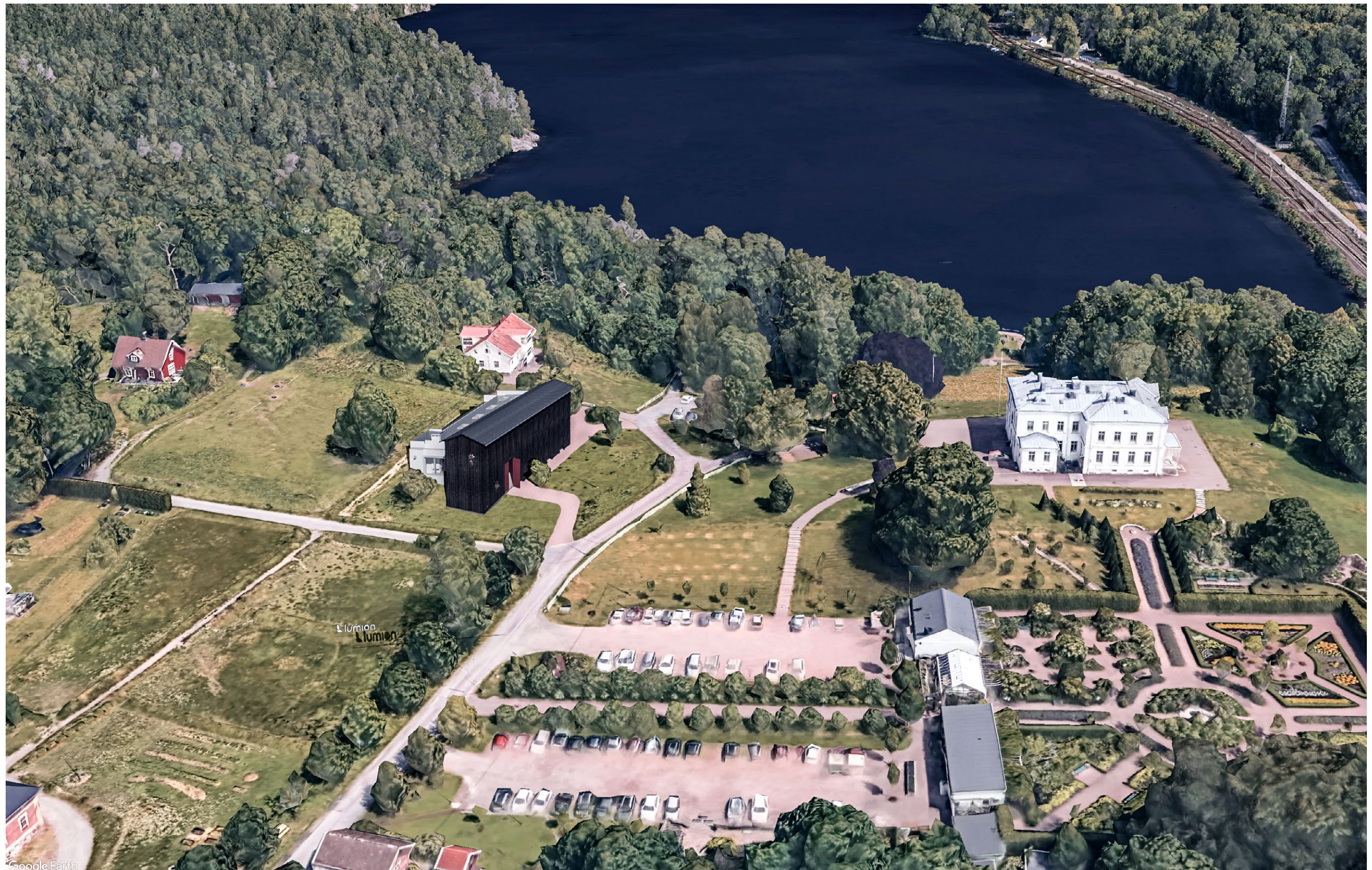
Fig 21. Overview of site and project.
