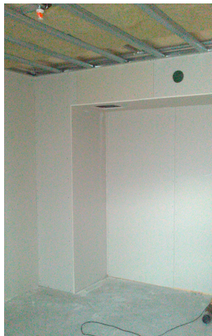
Figure 3.5.: Photo of the gypsum walls in the floor, which include structural parts as pipes or ventilation that could not be integrated in the F.E. model.
