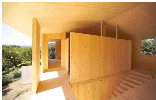
Figure 1.2.: Photo of a house construction with CLT [9].
