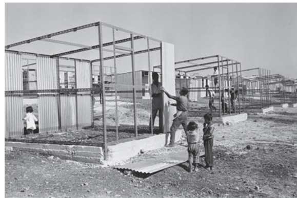
Figure 33, (Building the units, 1968, UNRWA Archive.)
