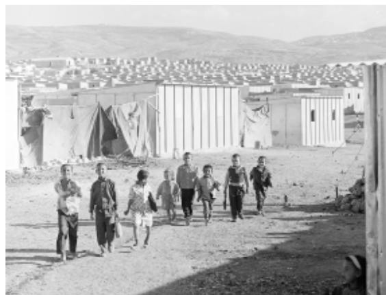
Figure 15, (Stage 3; prefabricated units, 1969, UNRWA Archive.)
