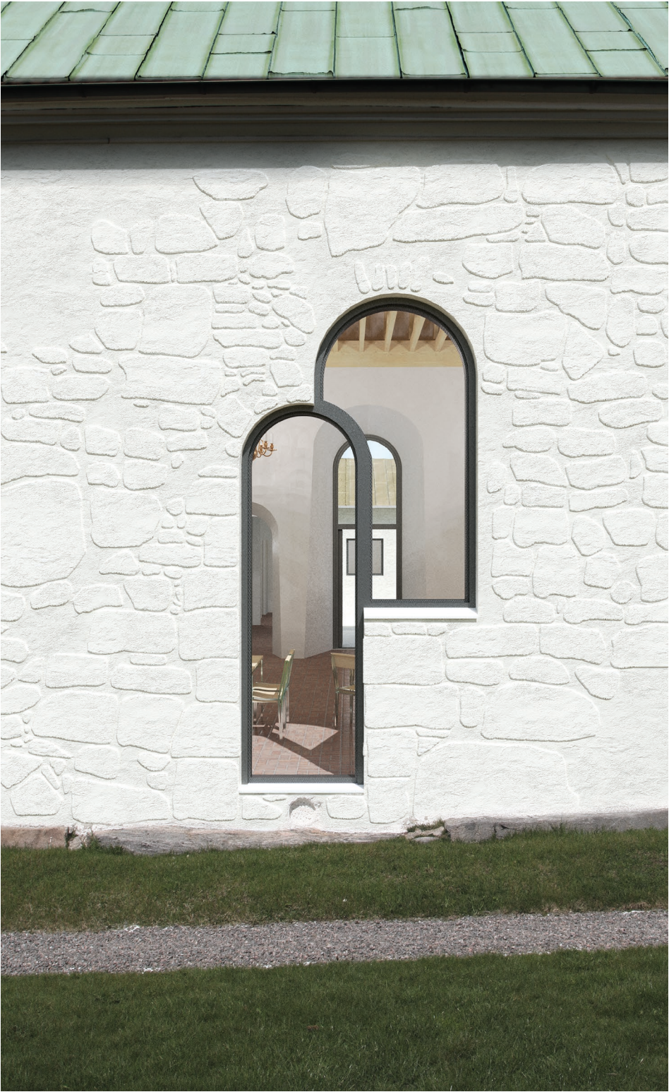
Fig. 97 View through the reopened south portal through the nave.
