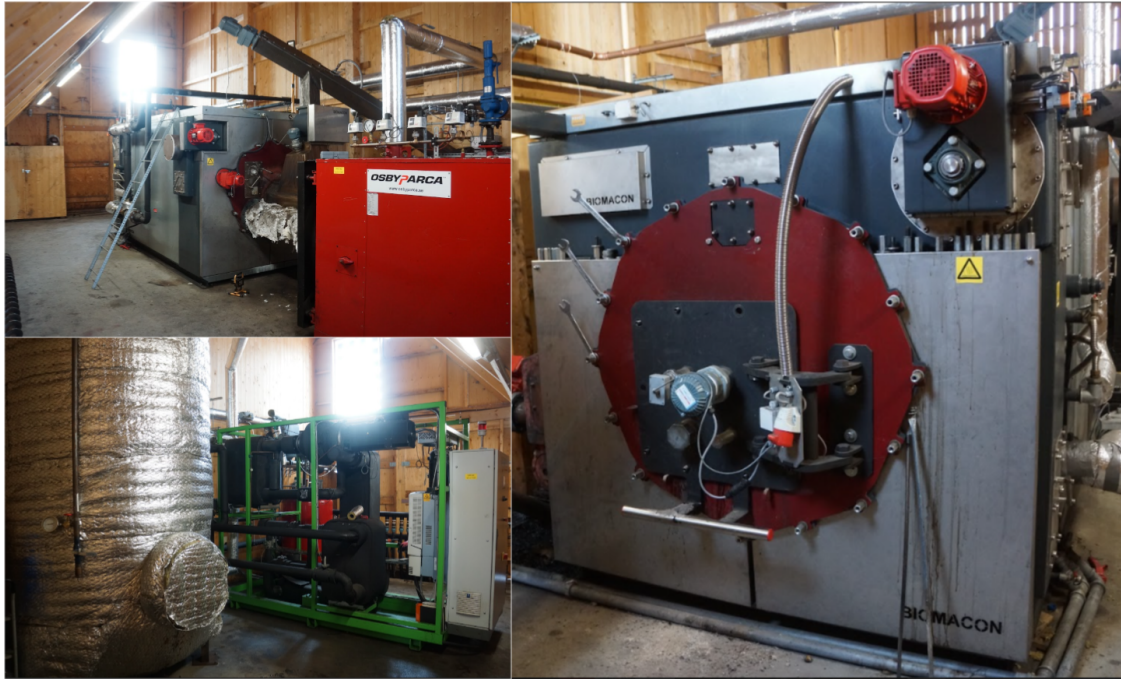
Figure 2.3: Picture of a pyrolysis plant package, delivered by Biomacon, for farm scale applications.
