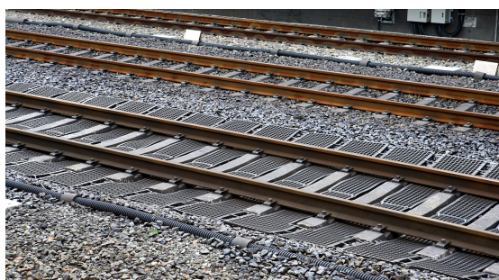
Figure 3.3: Shows a ballast mat that is used as a mitigation strategy close to the source. Note that this is a surface line. Source: Wikimedia Commons.
