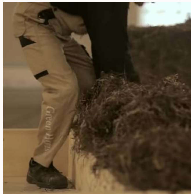
Eelgrass insulation in prefab wall. Image source: Realdania By & Byg, 2013
