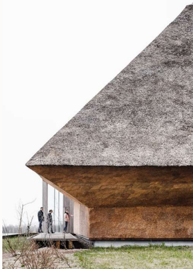
Thatched facade at Wadden sea center. Photograph: Rasmus Hjortshøj
