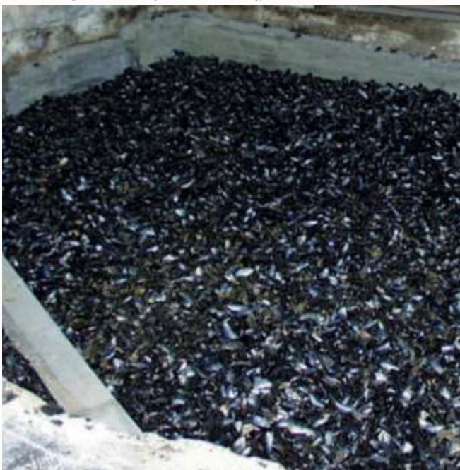
Mussel shell drainage in foundation. Image: Bondegaard Rydbjerg
