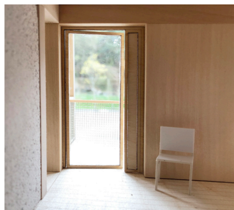
Model picture of vertical ventilation flap, steered by indoor air quality measuring device.
