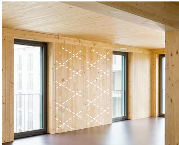
Figure 17. Dowel laminated timber structure in residential building, Haus J, Zurich (Spoerri, 2014).
