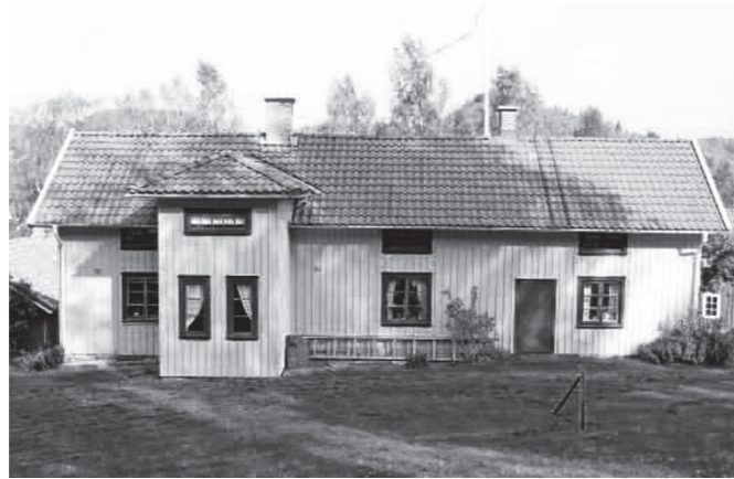
Figure 15. Unheated extension concept of a vernacular Framkammarstuga. The entrance to the heated part of the house works as a buffer zone (Hansen, Nordström, 2007).
