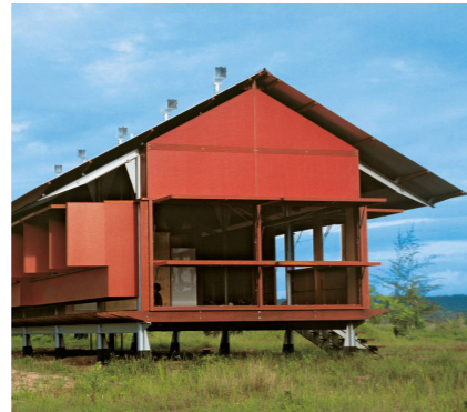
Figure 5. Marika-Alderton house. Glenn Murcott, Australia 1994 (Murcott, 1994).
