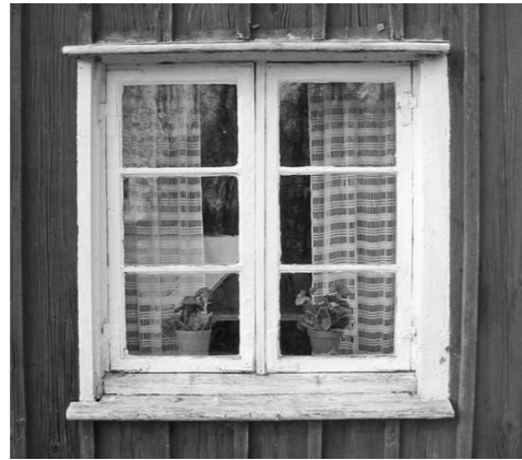
Figure 13. Single glazed window with interior winter pane. Air is warmed between the panes before it enters the dwelling (slöjd och byggnadsvård, 2021)
