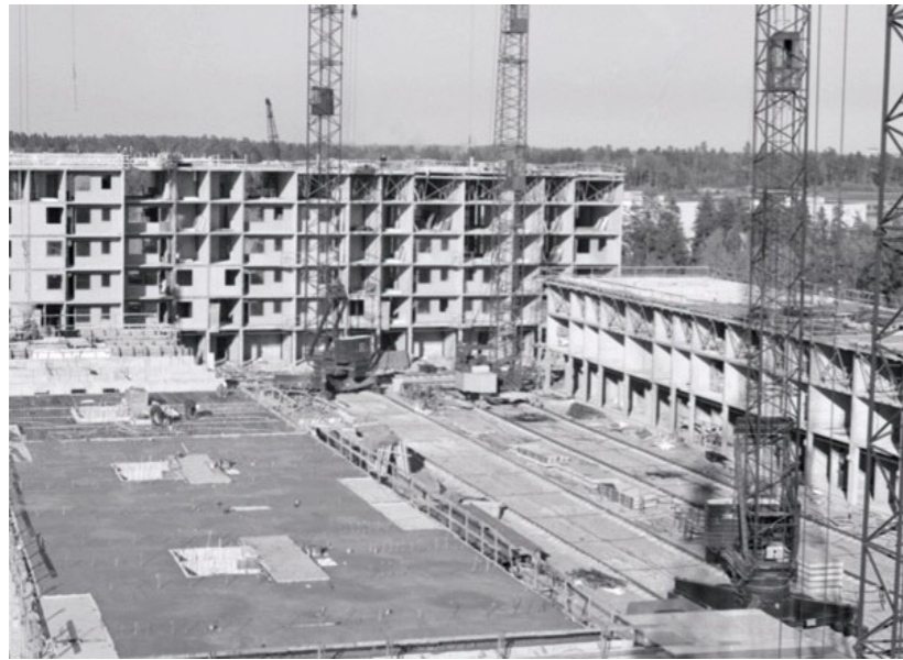
Figure 3. Construction of Hallonbergen, Sundbyberg (Gösta Nordins arkiv, 2021).
