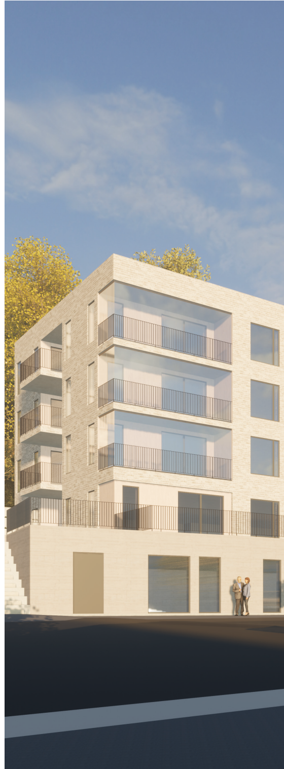
Figure 56. Corner of building
