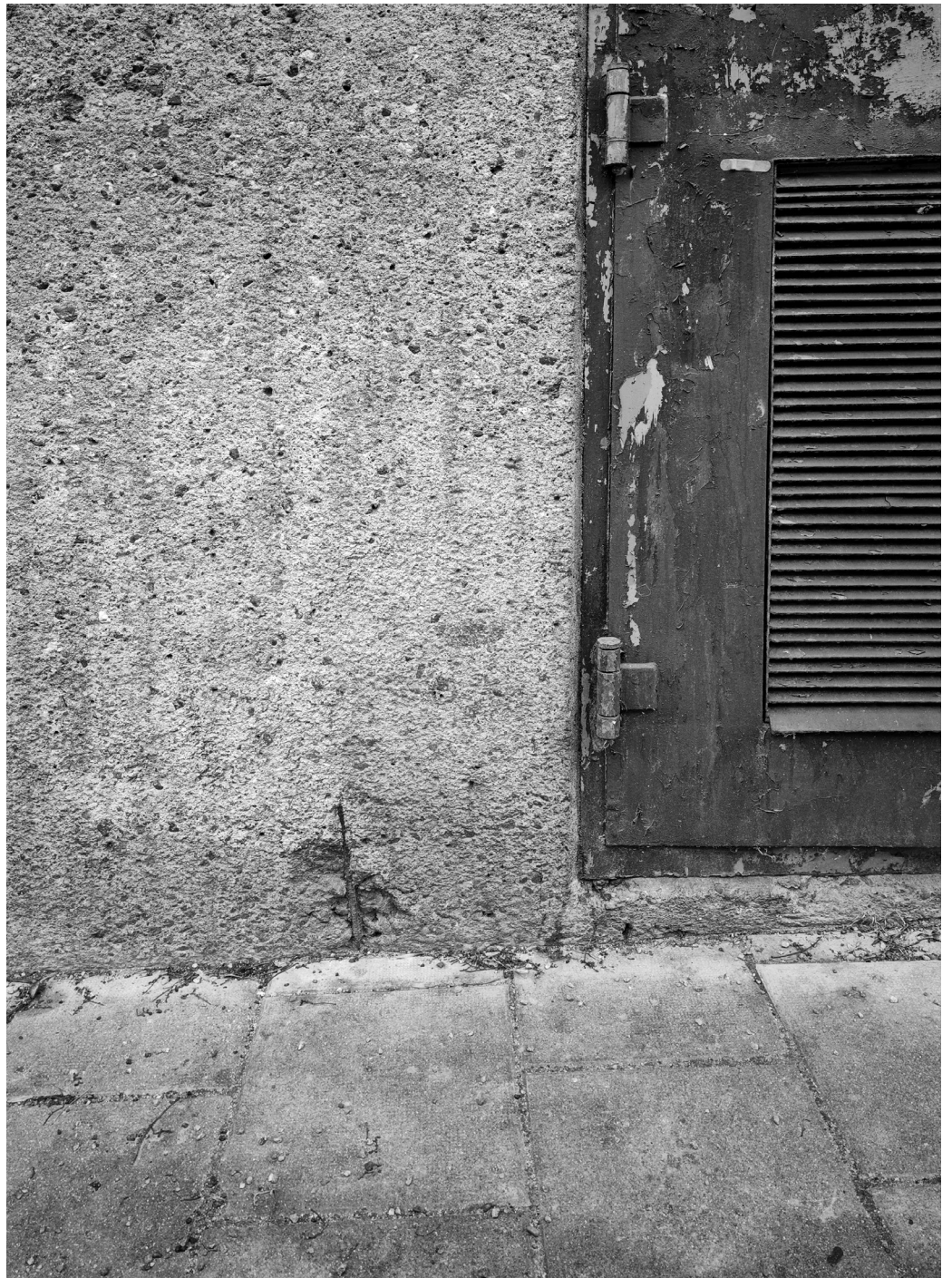
Fig.40 Damage of the reinforced bars, the concrete coating and deterioration of doors.
