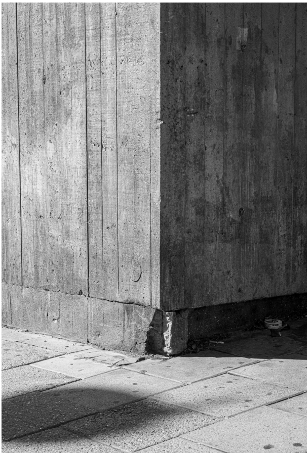
Fig.35 Trace of ageing, concrete crack. © Inès Romy
