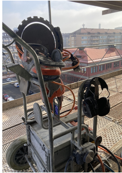
Figure 30: A power cutter transported on a carriage
