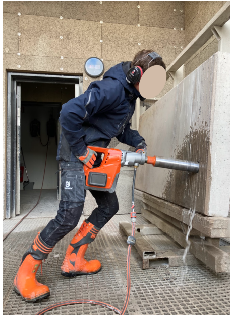
Figure 29: Picture from an observation showing how the core drilling machine is being supported on the user's thigh
