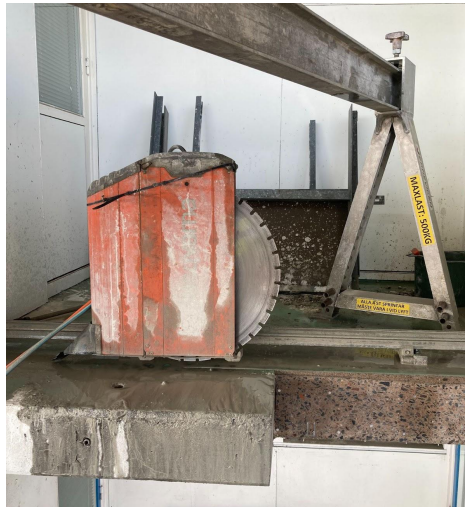
Figure 34: A wall saw attached to the floor
