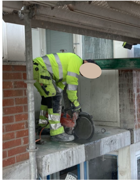
Figure 33: Cutting in the floor
