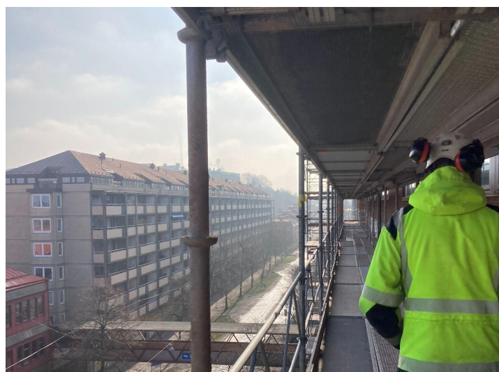
Figure 20: During one of the observations, walking on the scaffoldings
