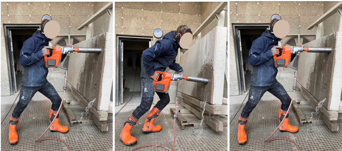
Figure 13-15: The three analyzed body positions for the core drilling machine
