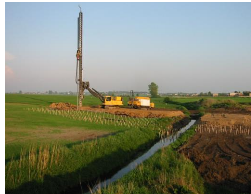
Figure 6 Column installation (Alén et al., 2005a).
