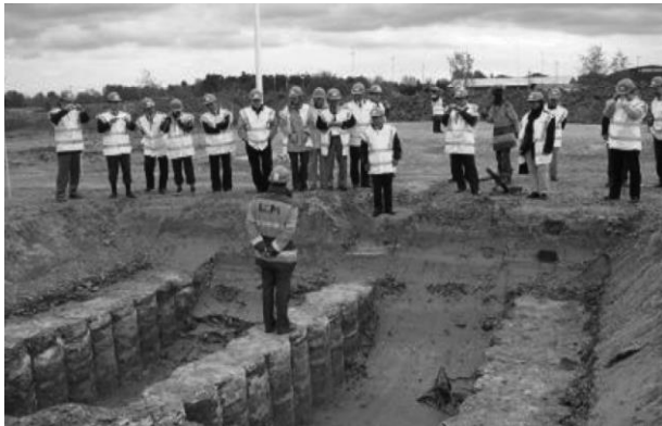
Figure 7 Interlocking Columns in Panels. Upsala, Sweden (Kirsch et al, 2012)
