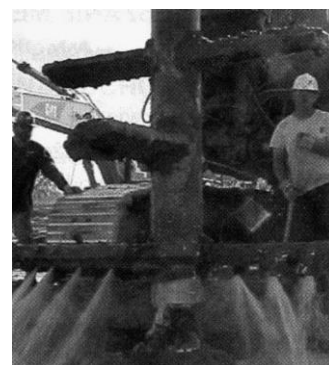
Figure 2 Typical wet mixing tools. (Topolnicki, 2003)
