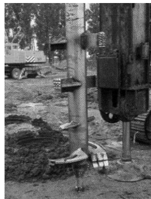
Figure 2 Typical wet mixing tools. (Topolnicki, 2003)
