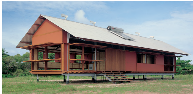
Marika-Alderton house Australia, 1994 Architect Glenn Murcutt
