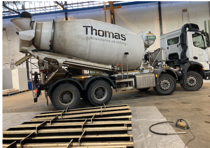
Figure A.7 The fresh concrete was poured into the forms from the concrete mixer truck.
