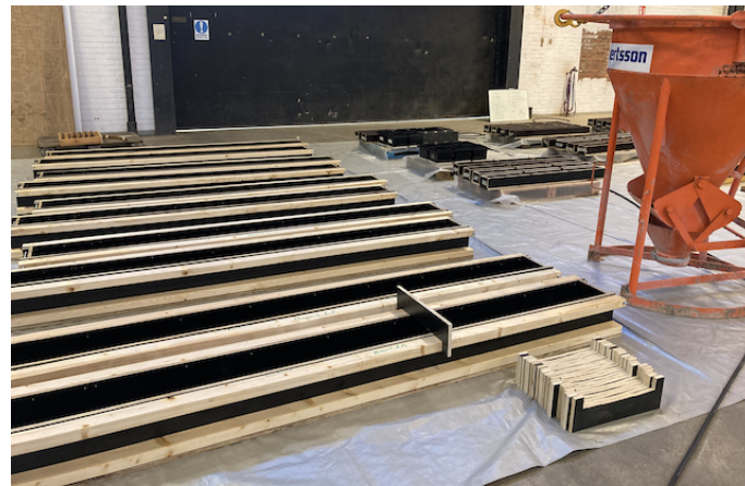
Figure A.6 Preparations of the forms before casting. The forms to the left were prepared for this thesis.
