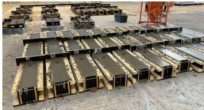
Figure A.8 Casting of the concrete beams.
