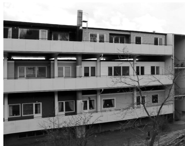
Figure 16. Kallebäck Experimental Housing in Gothenburg. Stacked "villas" in a concrete structure.
