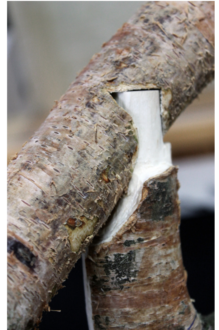
Fig. 66. Close-up of milled connection.
