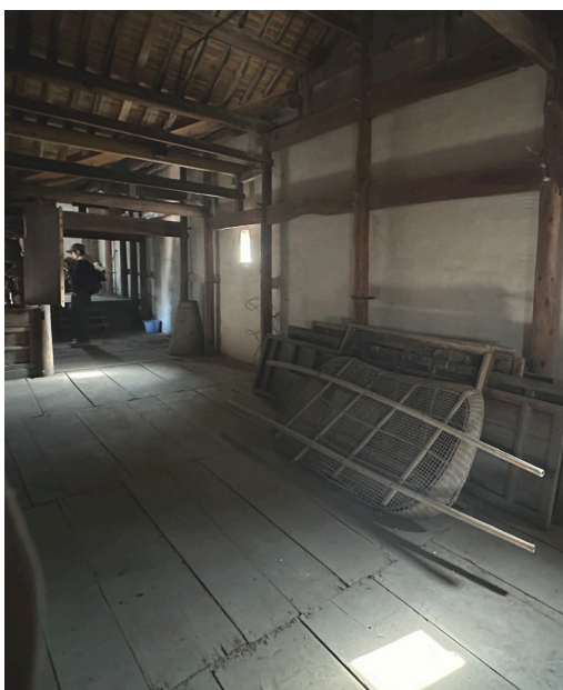
Fig. 24 Damaged first floor slab
