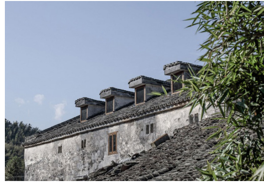
Fig. 52 Clerestory windows were added to the roof(Wang, R., 2018)
