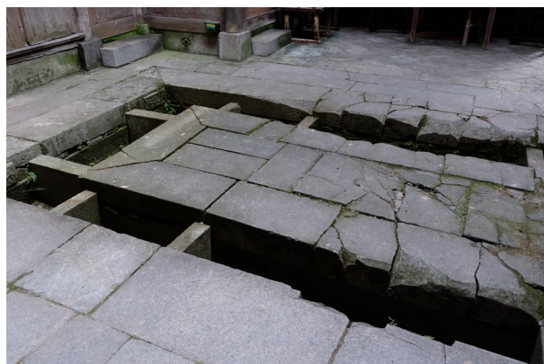
Fig.12 Ditches in courtyard
