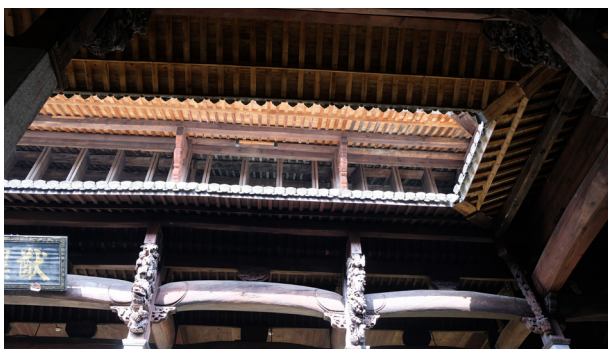
Fig.11 The upward view from courtyard
