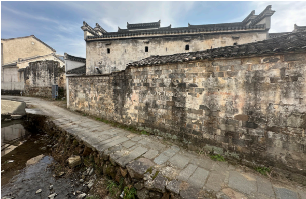
Fig. 38 View from river side
