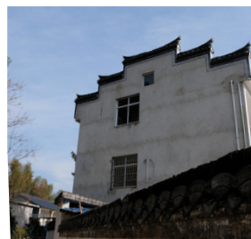
Fig. 42 Newly built residential buildings with modern features
