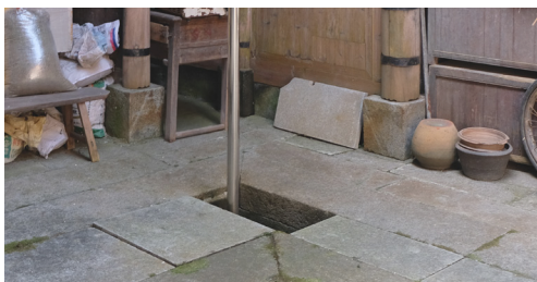
Fig. 23 New drainage pipe
