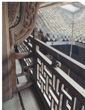
Fig. 18 View from the first floor (Beauty Lean)
