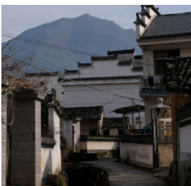
Fig. 41 Newly built residential buildings with modern features
