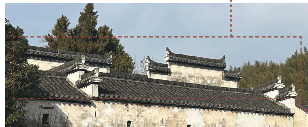
Fig. 25 View of eastern side of the building
