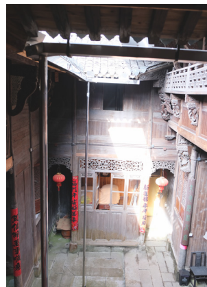
Fig. 26 View of the courtyard from the first floor
