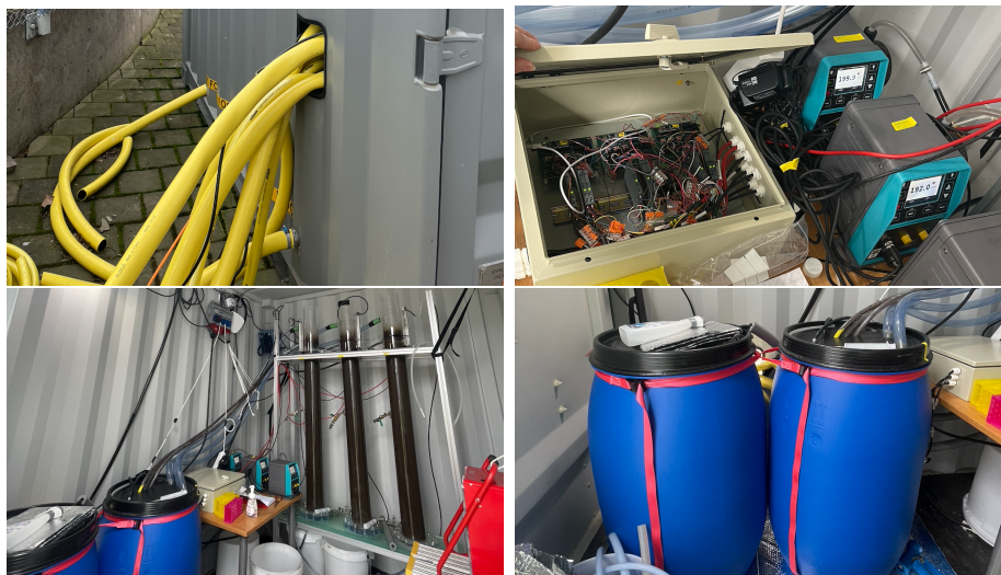
Figure 3.1: Pictures of how the pilot is constructed showing the hose system, arduino box, reactors and buffer tanks.
