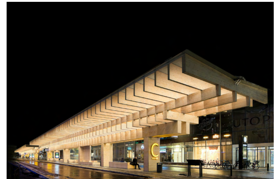
Image 18. Bus station in Umeå, designed by Wingårdhs. The illuminated over-dimensioned glulam elements lights up the otherwise dark and cold environment.
