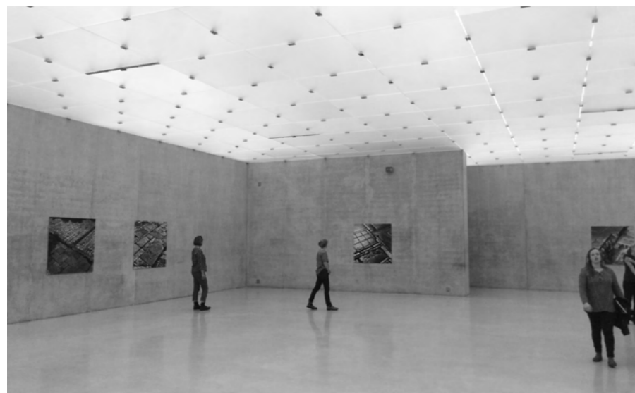
Room defining, stabilizing lamells
