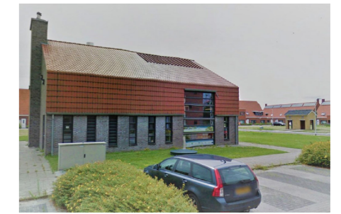
Figure26. Noorderhoek (Site: Sneek, the Netherlands)
